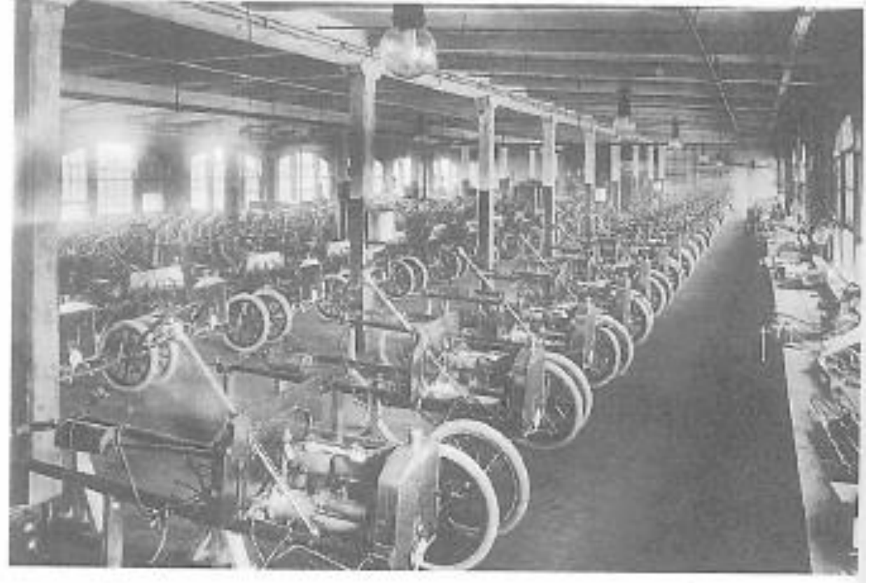
Assemble Box Production (old)
